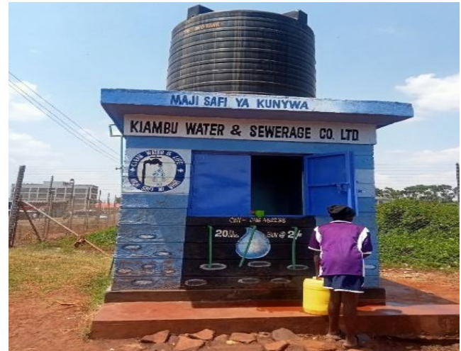
Photo 4: Water infrastructure in Ruturo (2024)
