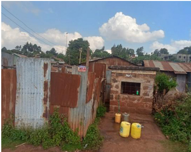
Photo 3: Water infrastructure in Kanjeru (2024)
