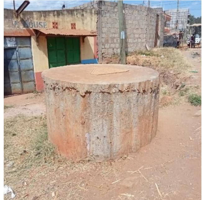
Photo 6: Sewer system seen at Madharau
