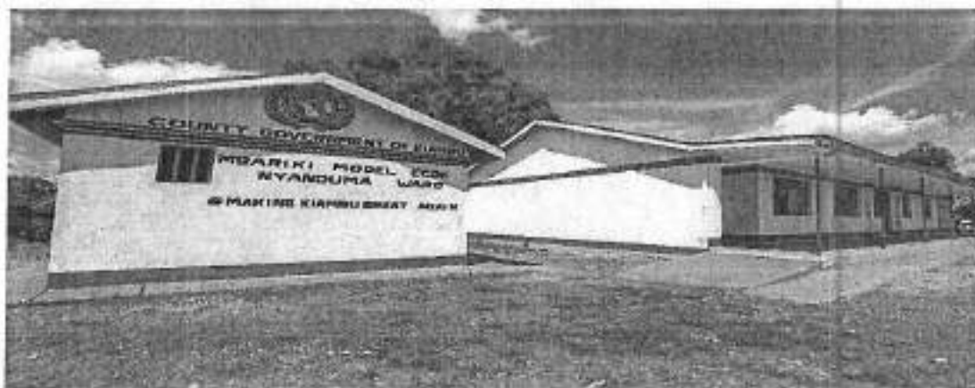
A newly constructed ECD Centre in Nyanduma Ward, Lari Sub County
