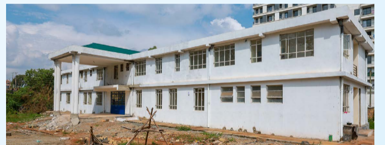
Ndenderu Level Three Hospital in Ruaka.
