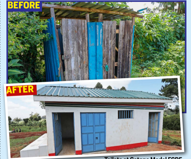
Toilets at Gatono Model ECDE Centre, Cianda Ward.
