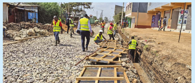
Ongoing construction of road in Gitambaya in Ruiru Sub-County.
