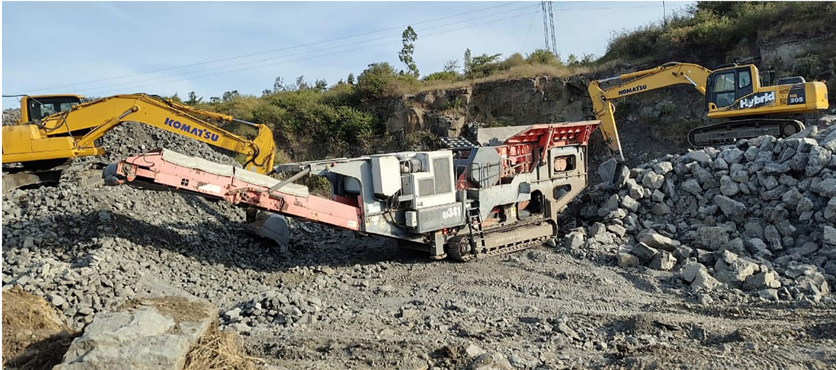
Ongoing excavation and crushing of rock boulders into hardcore chipping materials using Jaw Stone Crusher Plant at RUJWASCO Quarry/ borrow pit in Gatong'ora Ward, for roads rehabilitation and maintenance works throughout the County, to enhance mobility and accessibility.
