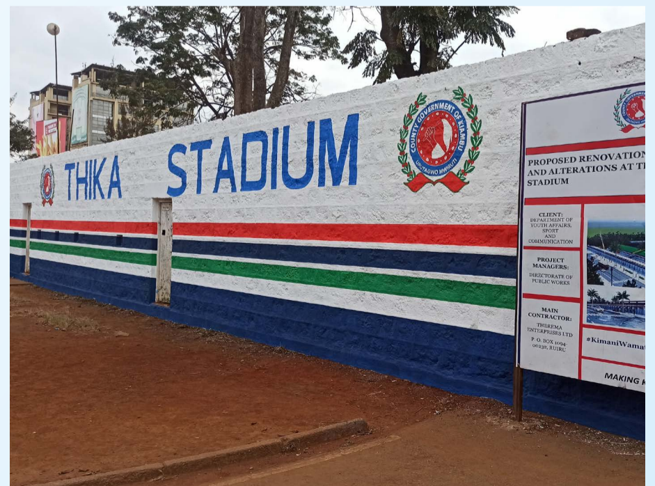
Ongoing renovations at Thika Stadium.
