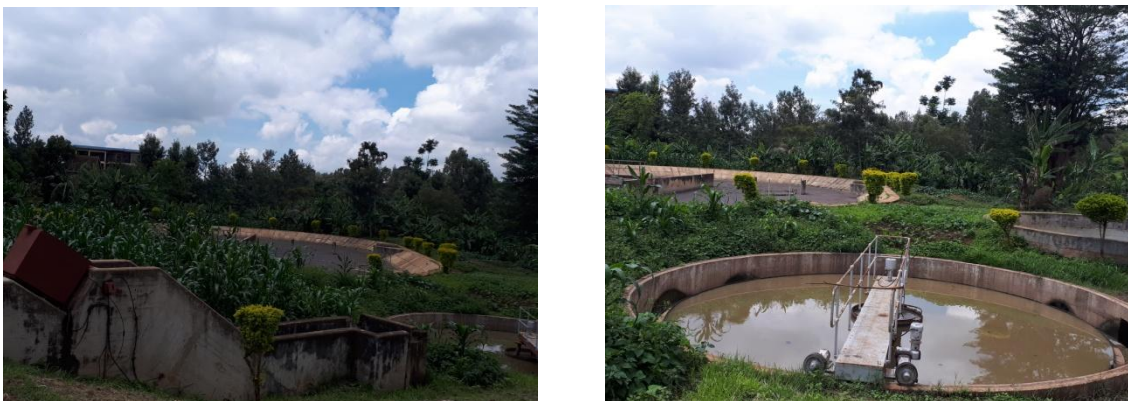
Figure 4: Limuru Sewerage Treatment Works
