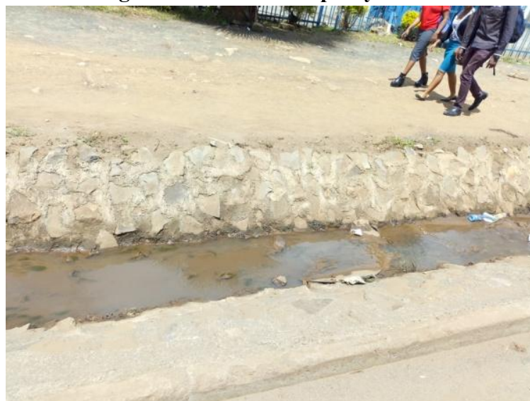
Figure 1: Storm Water Drainage in Limuru Municipality
