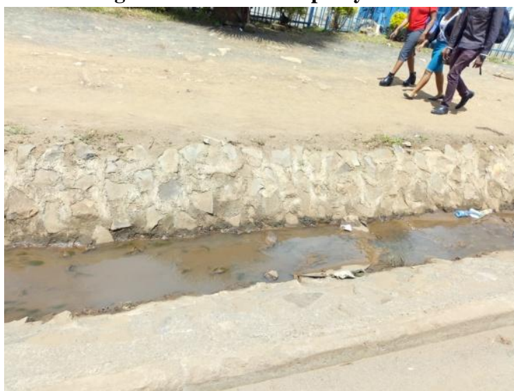
Figure 1: Storm Water Drainage in Limuru Municipality
