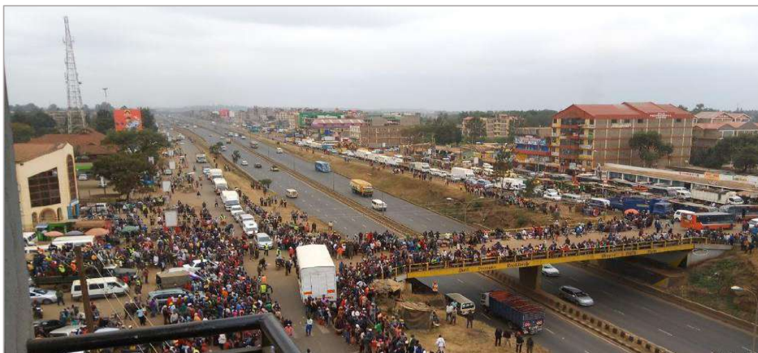
Figure 14-14: Shared vehicular and pedestrian overpass within Juja town
