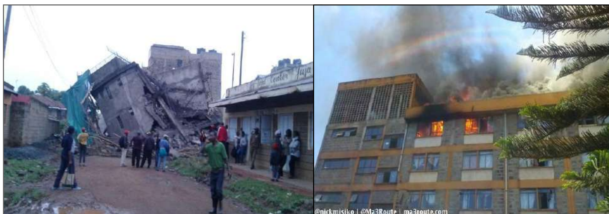
Figure 4-3: Collapsed building in Juja and fire outbreak
