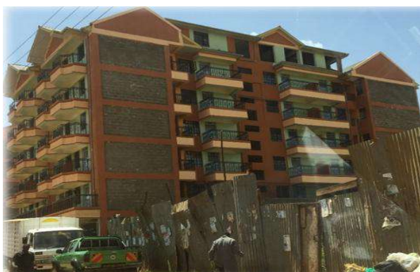
Flats in Gachororo
