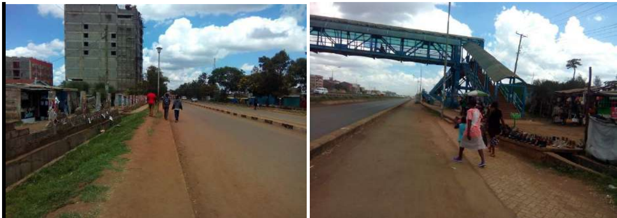
Figure 8-3: Poorly maintained footpath in Juja (Left). Footpath and a footbridge along Thika Super Highway (Right)
