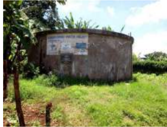
Riabai-Kihingo water project
