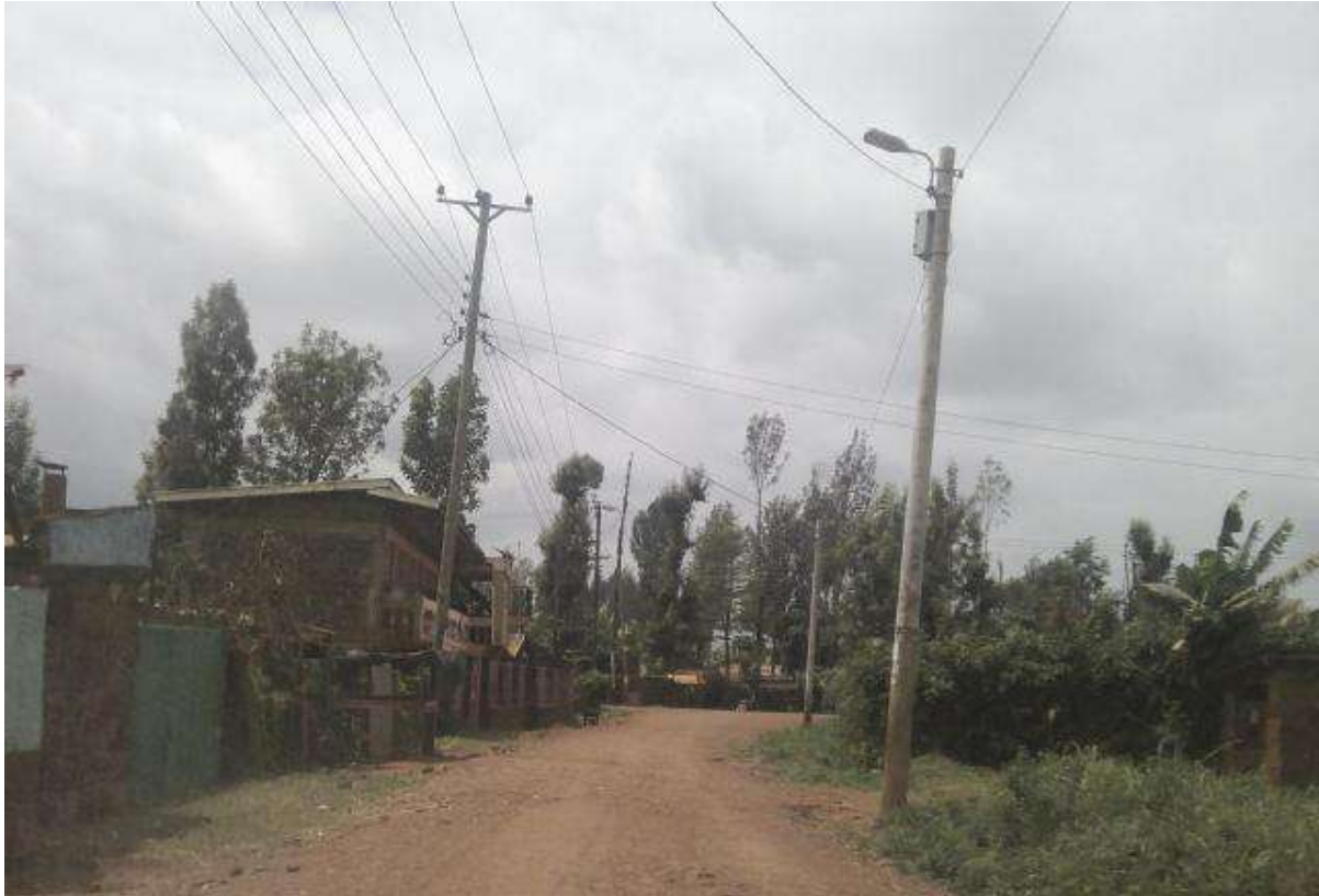
Figure 15: Power lines in Kiambu Town
