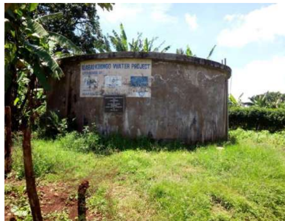
Riabai-Kihingo water project
