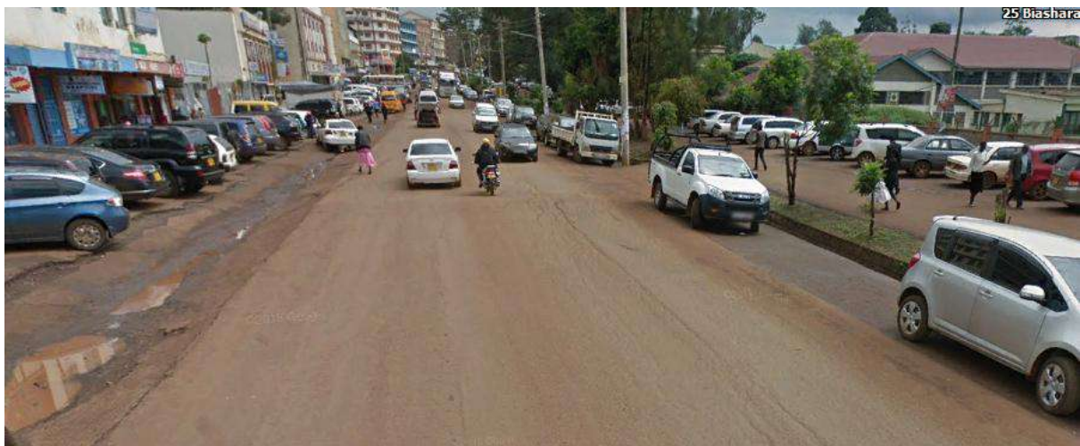
Cars parking on road reserves, insufficient storm water drainage.
