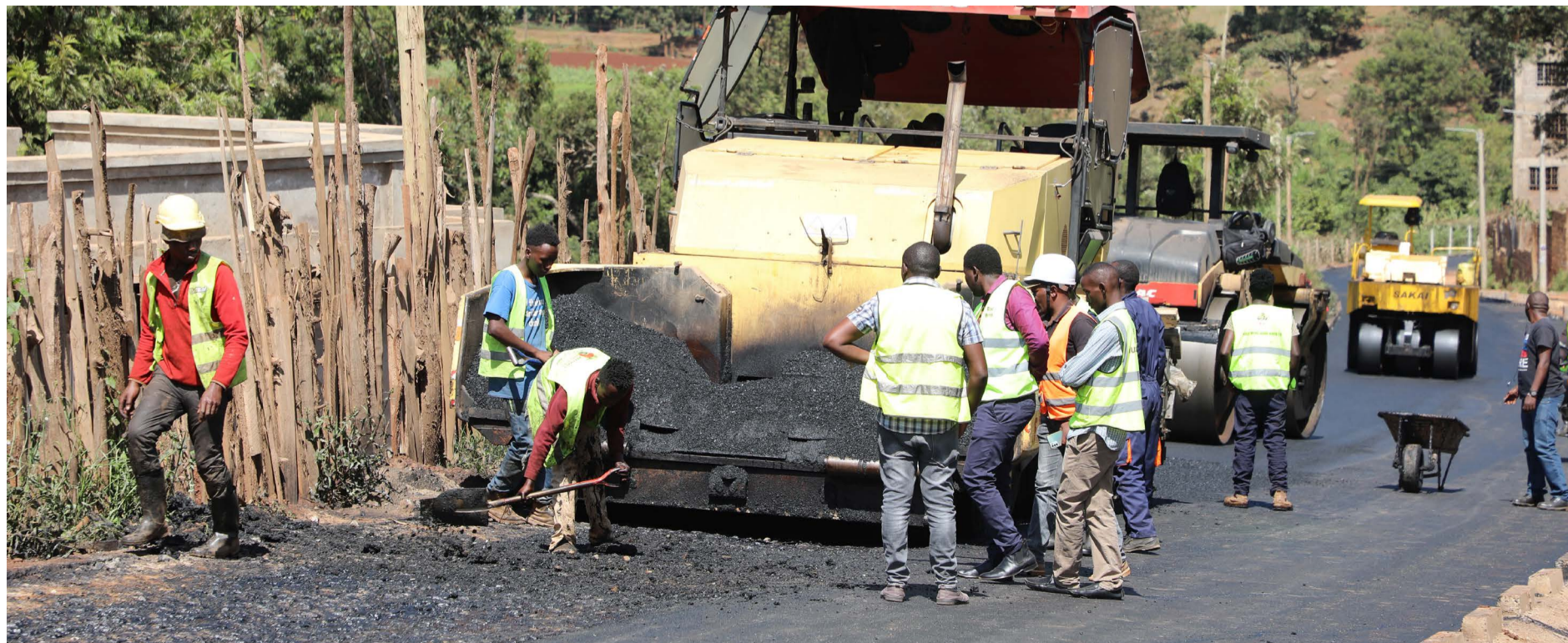
Tarmacking of Ondiri Road in Kikuyu.
