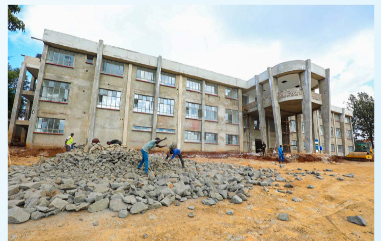
Thogoto Level Four Hospital in Kikuyu Sub-County
