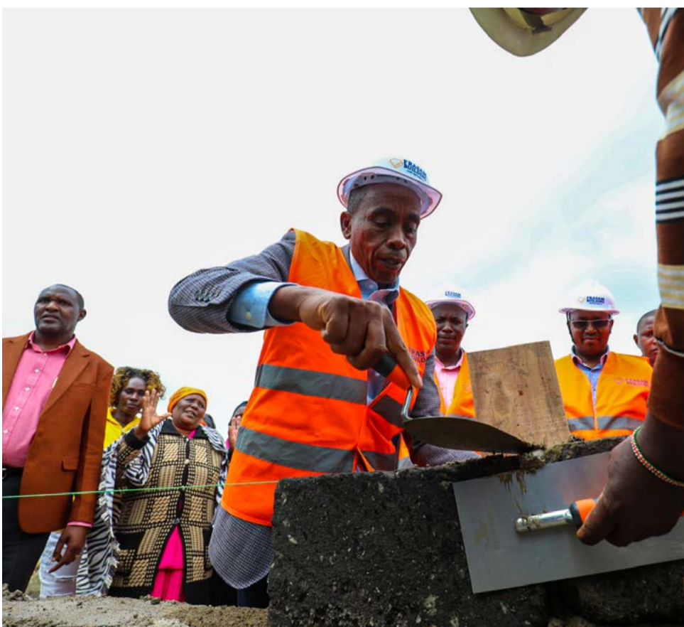
Commissioned the construction of Kimbo-Matangini Junction Market in Theta Ward in Juja Sub County.
