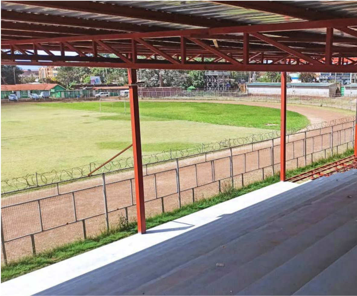
Ongoing construction of spectator stands at Thika Stadium in Thika Sub-County.
