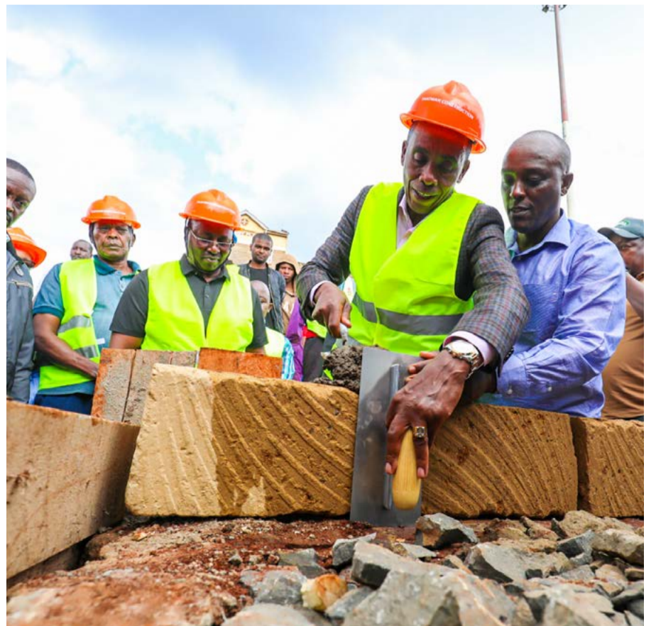
Commissioned the construction of Kinoo Market in Kinoo Ward, Kikuyu Sub-County.
