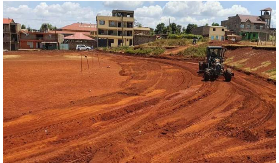
Leveling of Kanjeru Stadium in Kabete Sub-County by the Department of Youth Affairs and Sports.
