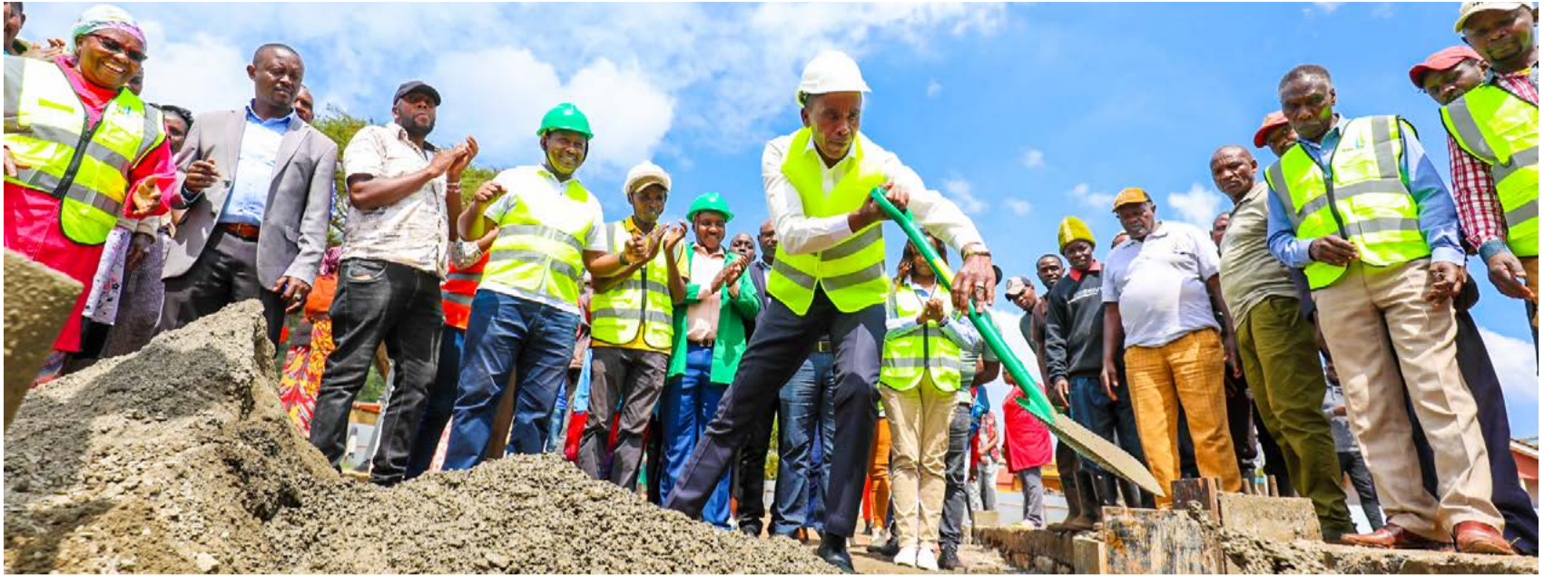
Inspection of the ongoing construction of Lusigetti Market in Nachu Ward, Kikuyu Sub-County.
