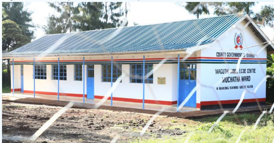
Waguthu ECDE centre in Muchatha Ward, Kiambaa Sub-County.
