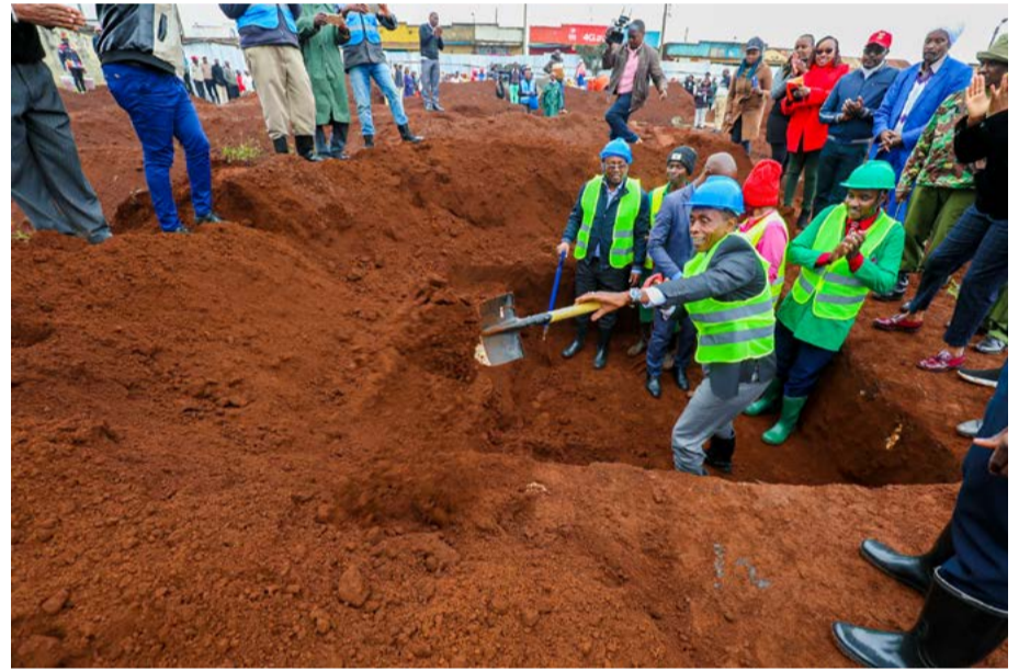
Commissioned the construction of Kagwe market in Nyanduma ward.
