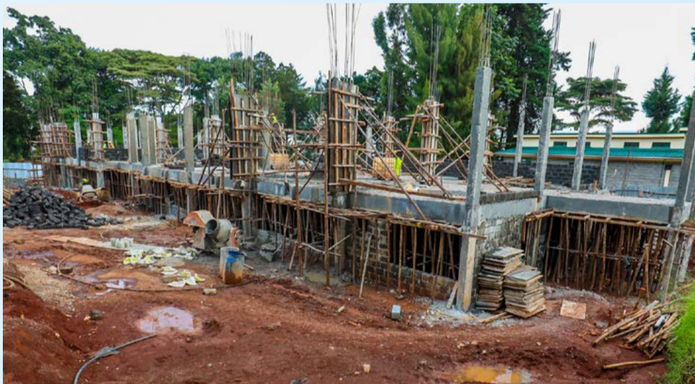
Ongoing construction of Karuri Level Four Hospital in Kiambaa Sub-County.
