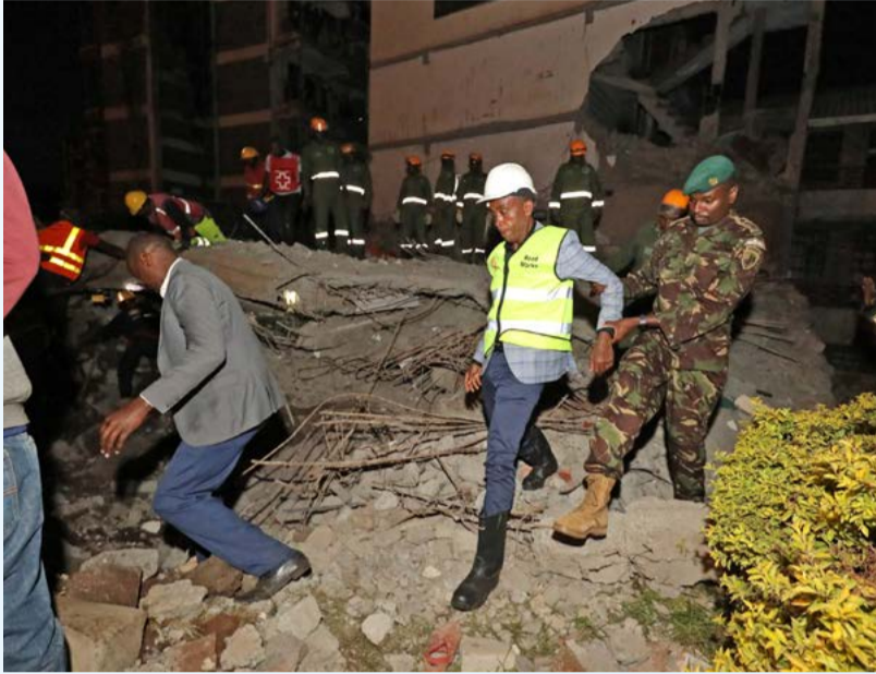
Governor Kimani Wamatangi at a collapsed building in Gitaru, Kabete Constituency
