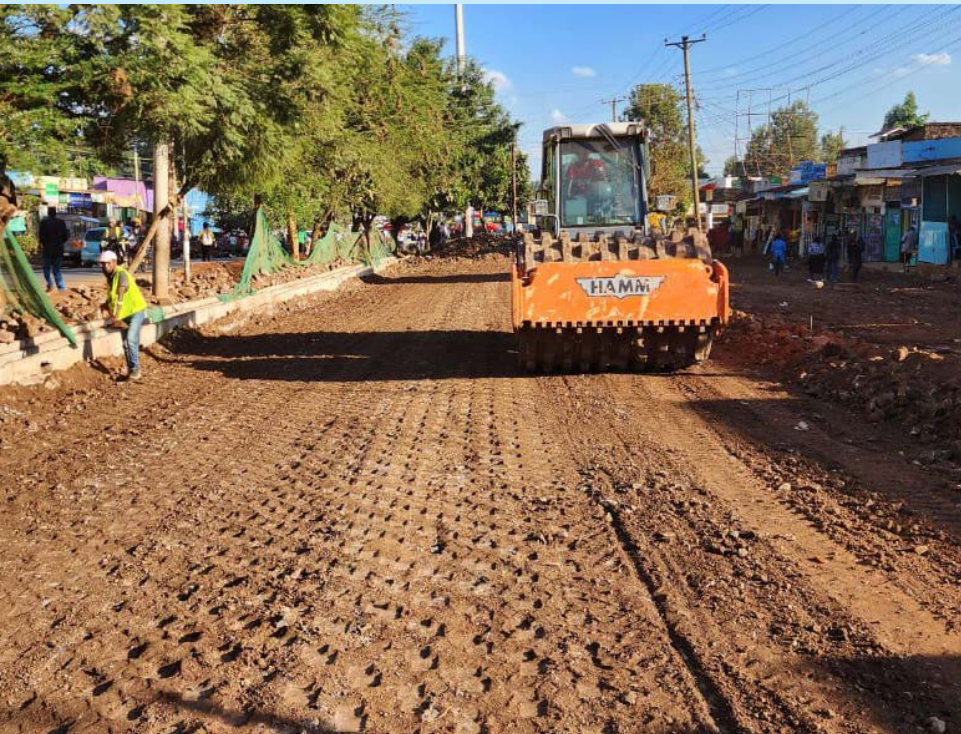
Processing sub-base on Banana bus park
