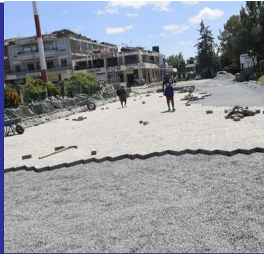
Cabro paving works around Felma Park in Kahawa Sukari.
